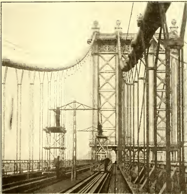
CATENARY TROLLEY CONSTRUCTION ON MANHATTAN BRIDGE—CONSTRUCTION GANGS ATTACHING HANGERS BETWEEN MESSENGER WIRE AND TROLLEY WIRE
